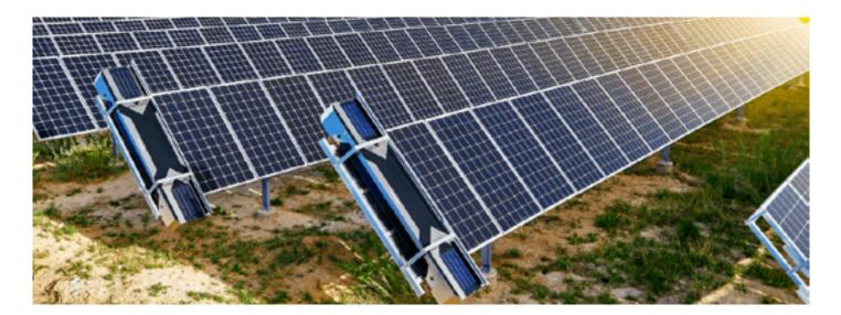
It is used to remove the dirt and dust deposited on the solar panel thus helping the solar panel to absorb the maximum quantity of energy.
