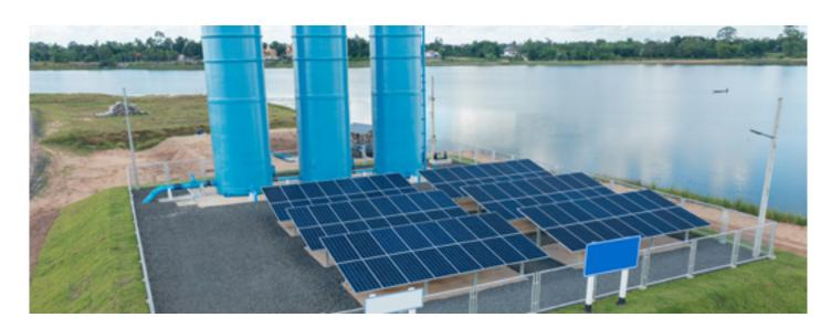
Solar water pumping systems are a common and essential use for solar photovoltaic modules. This Solar Pump drive may be used on any AC three phase pump, whether submersible or surface pumps, with the appropriate rating, and is developed using MPPT technology to enhance water delivery at different solar energy levels.
